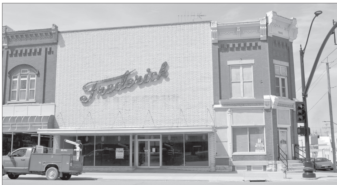
A project to renovate and add apartment units to the upper story of the former Frederick Furniture building has been temporarily stalled due to historic preservation standards, but work is expected to begin by January or February of 2019. (Michaela Kendall/The Grundy Register photo)
